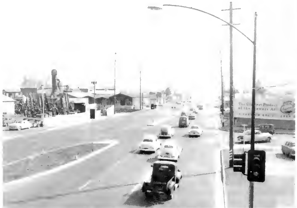
Looking south across the intersection of Union Avenue with Twenty-fourth Street
